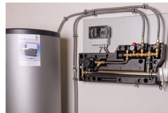
**heating insert to save costs. The latter requires a smart heating insert that can be combined with all commercially available energy managers / SmartHome / SmartGrid systems. Depending on the type, control is via relay circuit, WLAN / LAN, Modbus-TCP or 0-10 V.**
